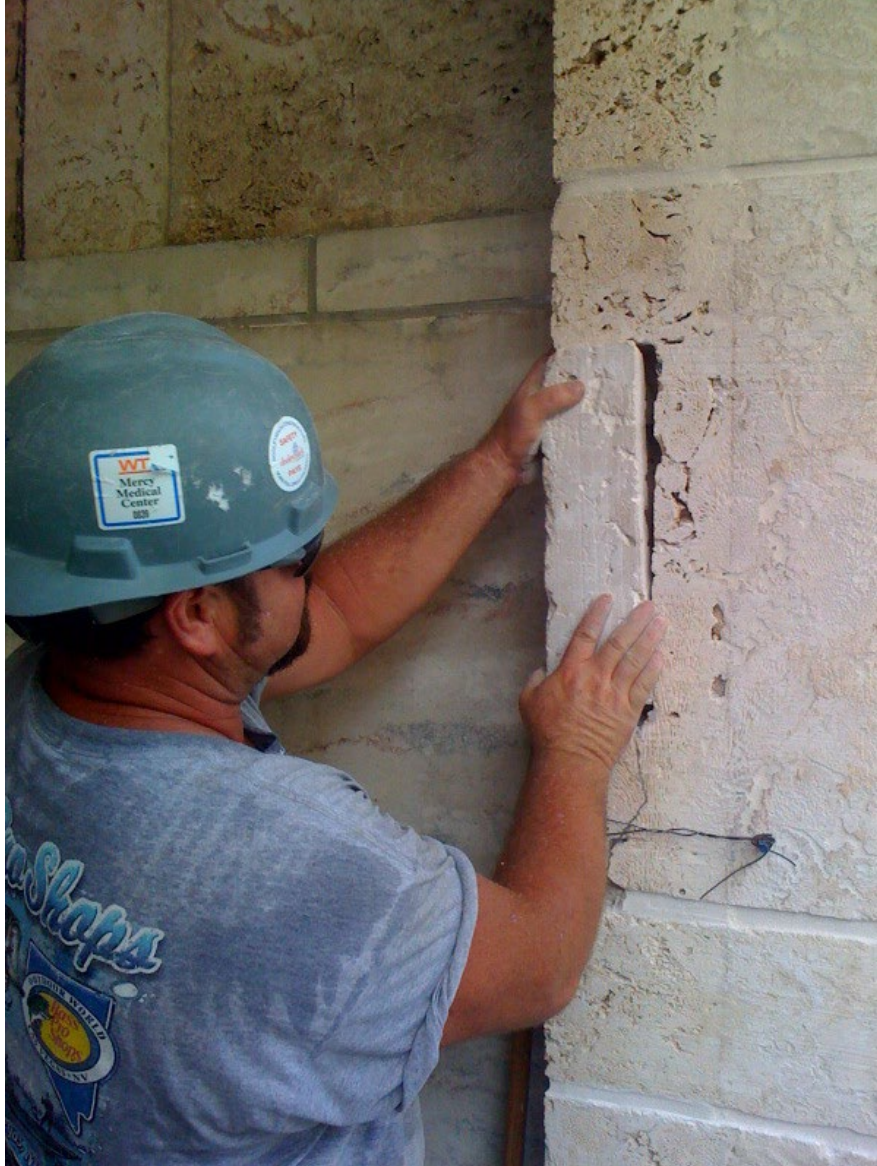
A mason works on repairing damaged oolitic limestone walls on historic building.
